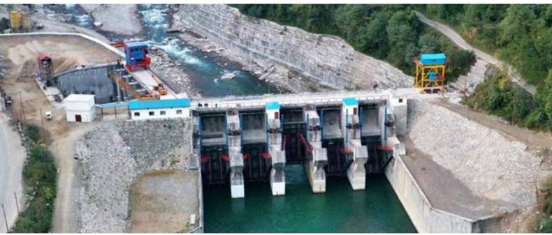
Barrage for Singoli-Bhatwari Hydro Electric Power Project (3x33 MW), Uttarakhand
