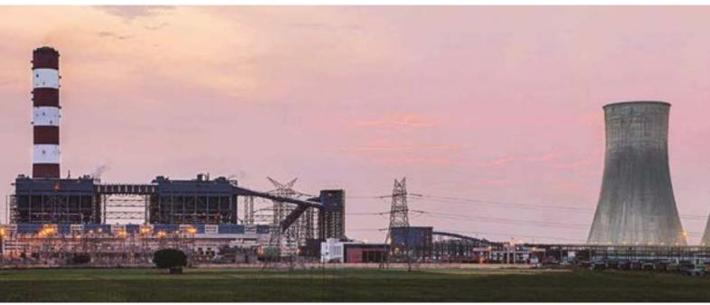
2x700 MW Supercritical Technology based Thermal Power Plant at Rajpura
